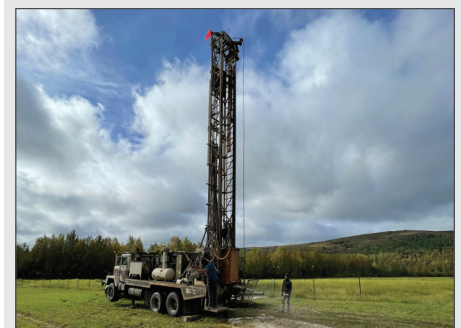
We are working with a drill rig to find and drill through the entire permafrost table. Our deepest borehole to date was 55 m.
